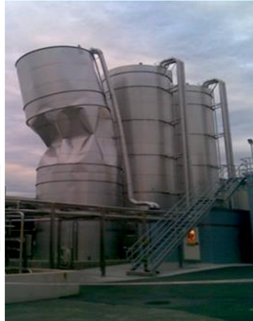
Voilement d'une surface comprimée in Coupling Experiment and Nonlinear Numerical Analysis in the Study of Post-Buckling Response of Thin-Walled Airframe Structures, Tomasz Kopecki
